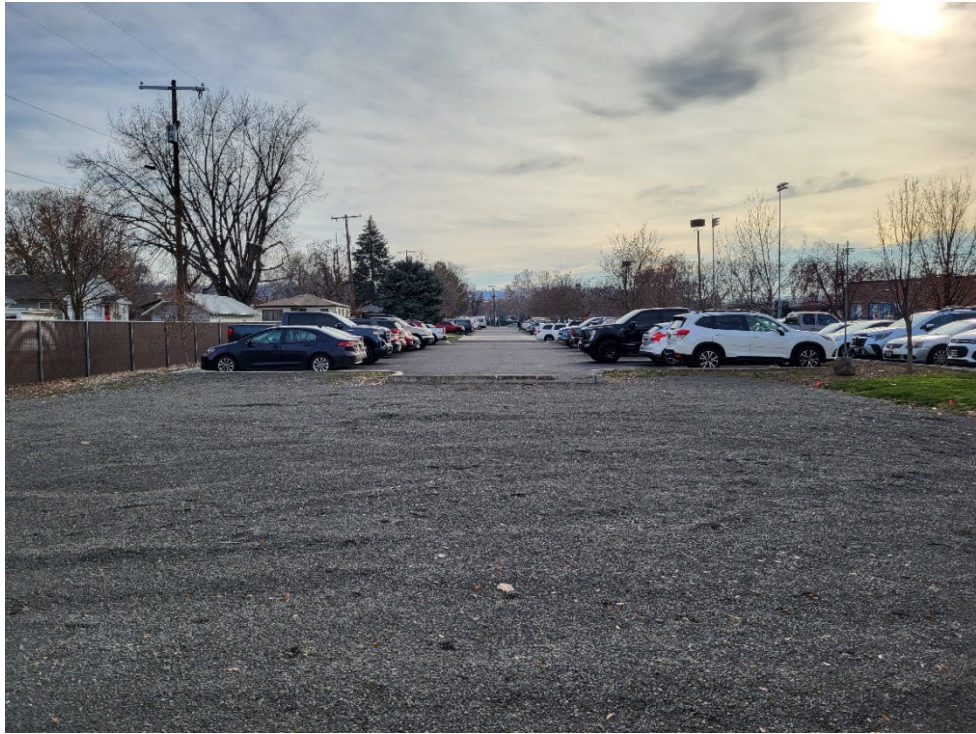
Northeast section of existing parking lot, location of demolished 4-plex apartment (foreground)
